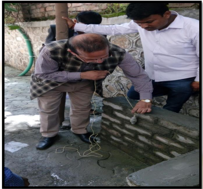
Checking quality of work
